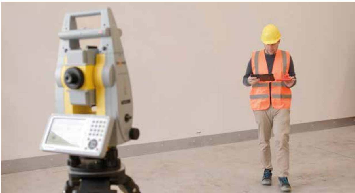
Staking out with the Stake Out Aid for Robotic Total Stations RS150M*
