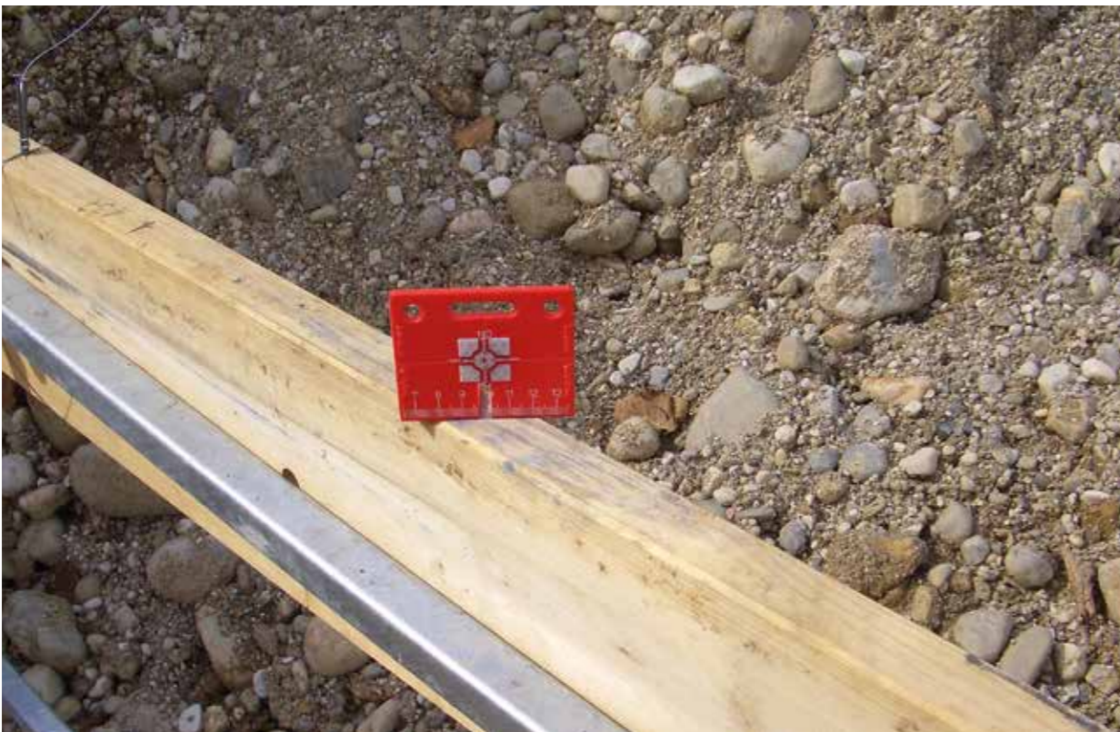
RS95 – Stake out work on the batter board
