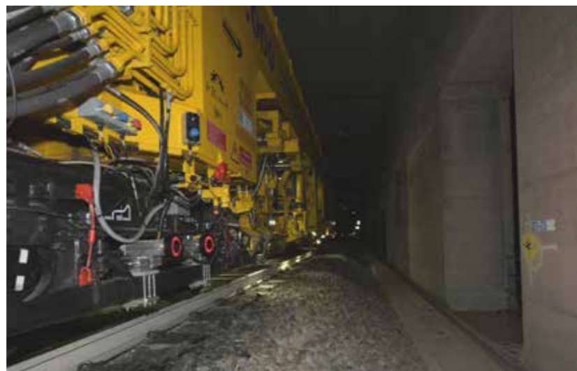
The RPM system installed on the 08-275 Unimat Combi (RFI Italia) tamping machine
