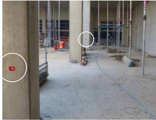
RS30r in industrial construction: documentation of heights and axes in one product.
