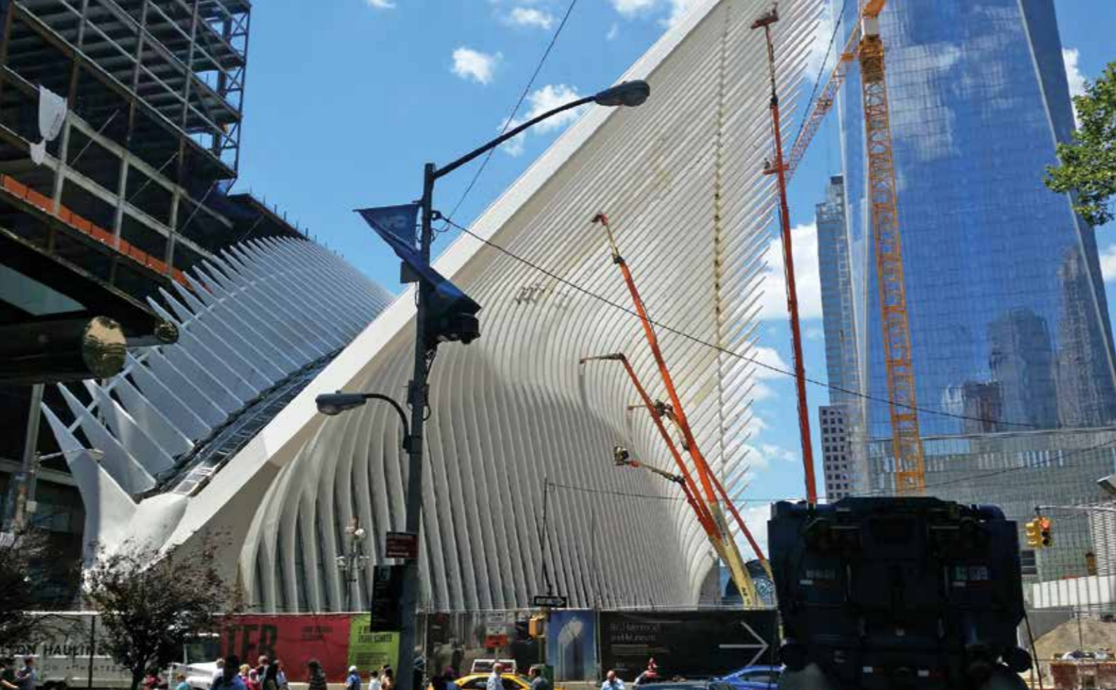
Subway Station, World Trade Centre in New York City
