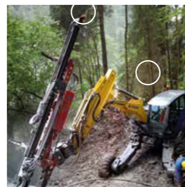
Example of the use of RS193M* as a fixed point on different surfaces and for the exact alignment of the drill carriage.
