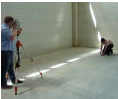
RS95 – Stake out work on the batter board
